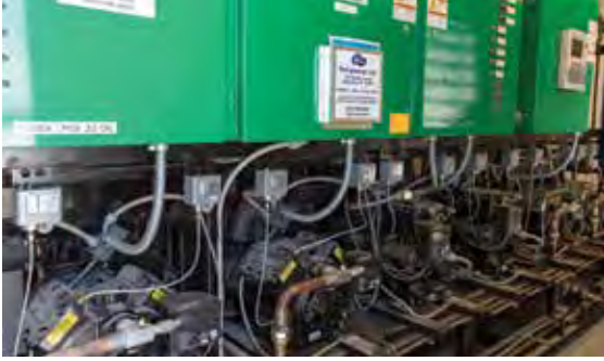
Medium-temperature rack designed for Solstice N40, manufactured by Zero Zone and maintained by John's Refrigeration
