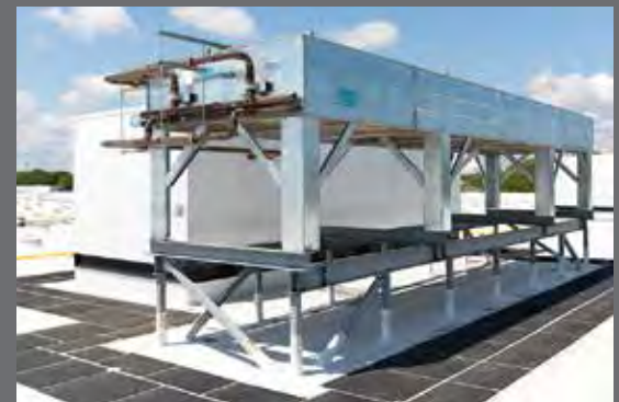
Medium-temperature roof rack house
