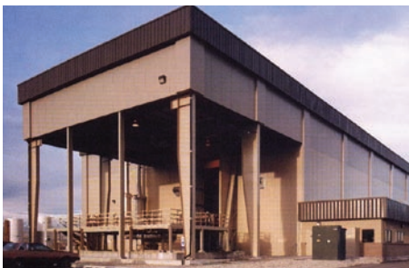
Salt Lake City Sodium-Reduced Sponge Facility
